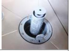
The grey plastic drain plug and filter cage MUST look like this or the water will not fill and the dishwasher will not work!
