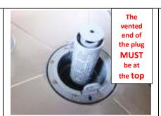
Ensure that the filter cage is in place and that the 'plug' end is inserted and pushed right to the bottom.
