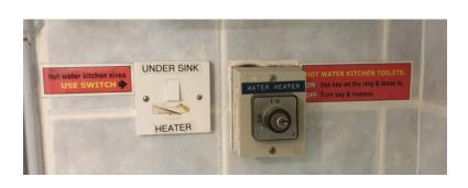
inserting the key on the hall key ring into the silver control and turning the control. To remove the key it is necessary to turn this water heater off.
