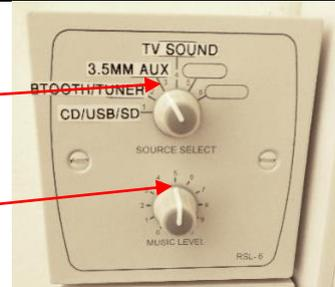
**2. Connect one end of the AUX cable to your Phone/Laptop/iPad and the other end to the jack socket on the wall below the selector switch.**
