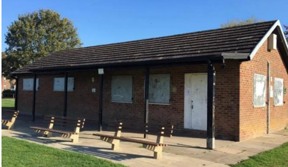
The old, not fit for purpose Pavilion.
